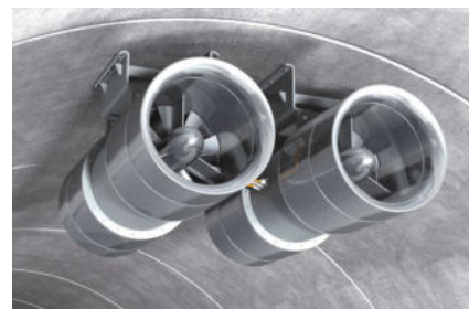
Wentylatory w tunelach
